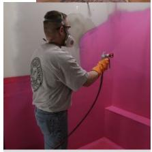
The use of spray equipment can greatly speed the installation of liquid-applied membranes on larger projects.
