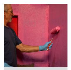
ANSI A118.10 not only assures that the membrane is waterproof, but that it has the strength to hold up for the life of the tile assembly.
