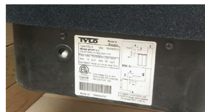
Resetting the temperature cut-out Temperature cut-out sauna heater
