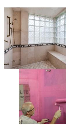
waterproofing in these spaces must be complete and monolithic. Unlike sheet-applied membranes, there are no cuts or folds to be made to fit into corners with bonding mortar. RedGard liquid can be rolled, troweled or sprayed on the surface for maximum efficiency and coats all surfaces and transitions with a continuous film.
