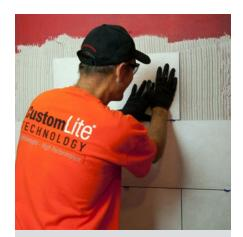
All tile in a steam room or shower should be installed with a dry-set cement mortar meeting the requirements of ANSI A118.15
