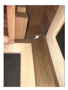
Firmly attach the 2-conductor cable to the open end of the LED strip. Give the cable a gentle tug to make sure the connector is locked onto the LED strip. Push the excess cable back into the wall cavity and secure the valance to the sauna wall with wood screws.
