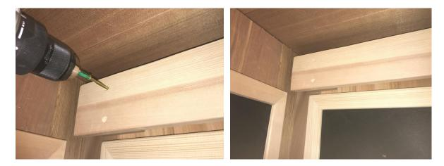
Attach Valance to wall with wood screws. Hint: mounting the Valance closer to the ceiling will give you less light wash on the ceiling. The lower you mount it, the more light wash you will have on the ceiling. You may want to turn the valance on and decide on the best position before securing to wall. Plug screw holes with wood plugs for a finished appearance.
