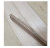
Nail and glue 1x2 strip over seam (on inside face of valance. Cut 2x2 provide to approximately 6" long pieces. Nail & glue as shown to ends and middle
