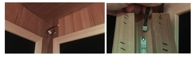
In this example, the Valance Light will be mounted on the back wall with the electrical connections in the left corner. Drill an access hole in the T&G paneling and feed the 2-conductor end of the special CAT5 cable to the center of where the 1x1 stand-offs will attach to the wall. You will need at least 6" of the 2-conductor cable to attach to the open connection on the LED strip. When mounting the valance you can push the extra wire back into the access hole.
