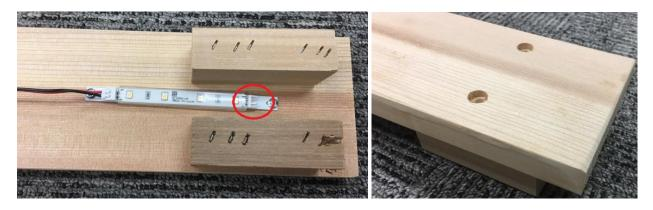
Either end of the Valance Light will have open contacts when all LED's are connected. The power cable from your 12vdc power supply or from your SaunaChrome Touch Control will connect to one of these ends. The other end can remain open. Attach completed valance to sauna wall by drilling/screwing through face of Valance and 1x1 stand off's.
