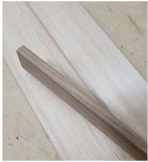
Nail and glue 1×2 strip over seam (on inside face of valance). Cut 2×2 provide to approximately 6" long pieces. Nail & glue as shown to ends and middle.
