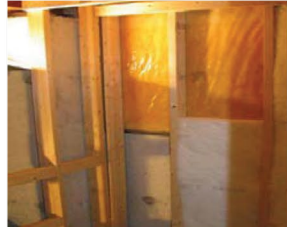
Cedar cleat (with kit) mounts through cedar lining into blocking.
