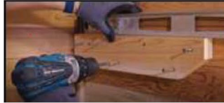
Cedar cleat (with kit) mounts through cedar lining into blocking.
