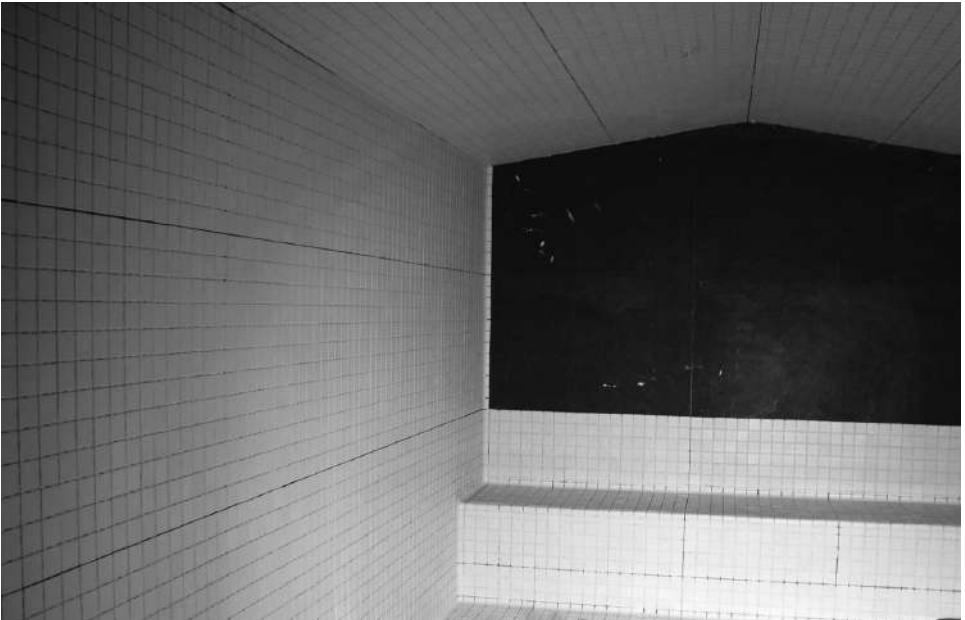
Continuing tile installation onto all surfaces using 254 Platinum.
