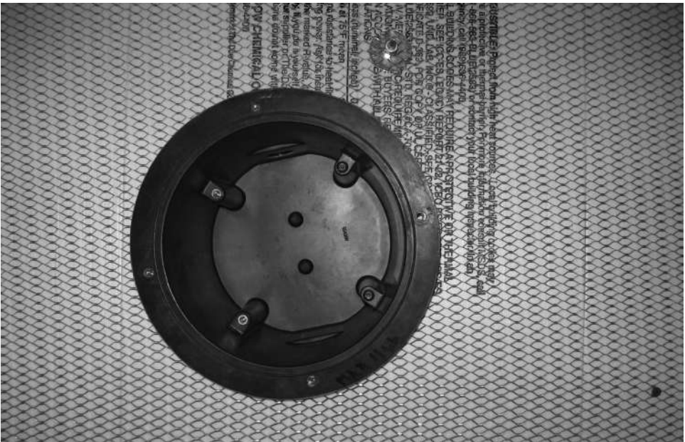
Tie-in of 3.2# expandable diamond metal lath to steam room light fixture.
