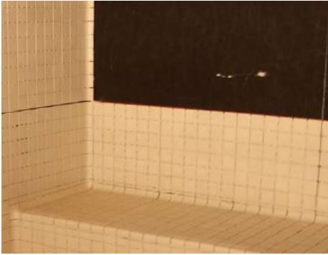
Figure 3.5.4 – Installation of tile in a steam room directly onto 9235 Waterproofing Membrane.
