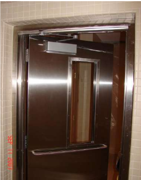
The finished tile installation and stainless steel steam room door.
