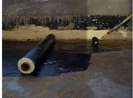
Figure 6.3.6 — 9235 Waterproofing Membrane applied to concrete substrate.
