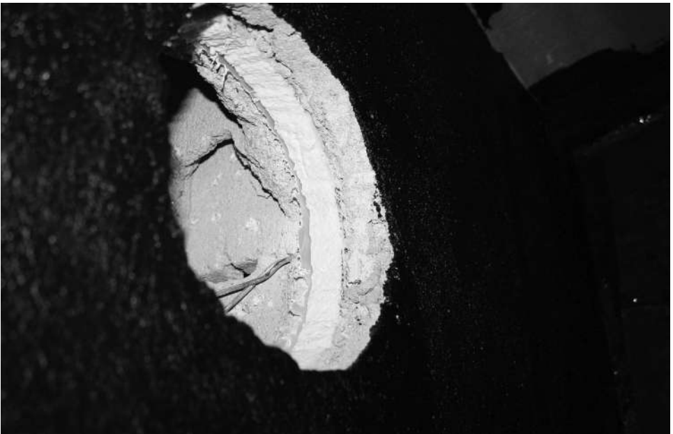
Scratching the 3701 Fortified Mortar Bed with a piece of metal lath.
