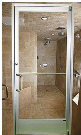
Figure 3.5.7 – Glass steam room door 22
